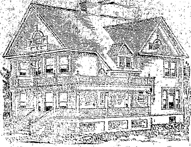
THE SUPERINTENDENT'S RESIDENCE AT THE NORTHVILLE U. S. FISH STATION.
